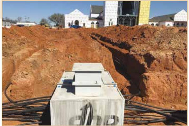
*Photo 4 – March 3, vault for valve manifold in geothermal well field, looking north, by Mark Pruitt*
