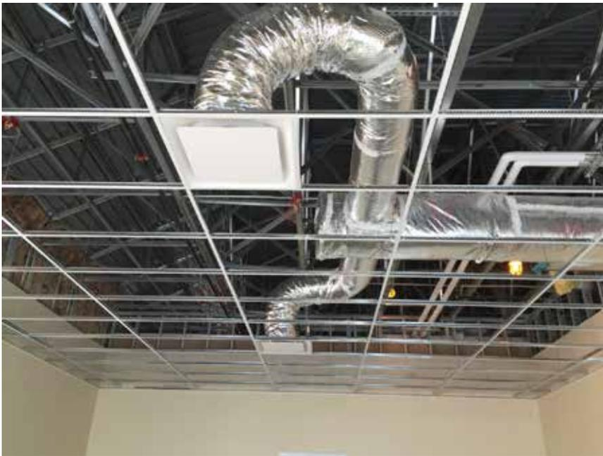
*Photo 2 – April 11, ceiling grid and HVAC diffuser installation in classroom, by Mark Pruitt*
